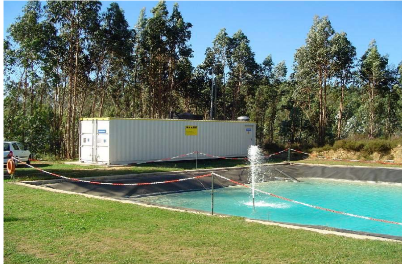
Plate 2.4: Typical configuration of a 2-stage RO plant with permeate lagoon (140 m 3 /d, Tondela landfill, district of Tondela, Portugal, commissioned 2004) (see Loeblich 2005)
