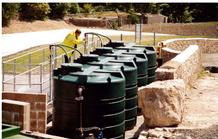
Plate 2.1: Typical methane stripping plant, treating up to 300 m 3 /d of landfill leachate, at Kendal Fell Landfill, Cumbria, 2002
