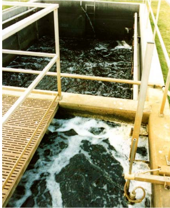
Plate 2.7: Typical reactor (35 m 3 ) for contact with PAC in treatment of landfill leachate
