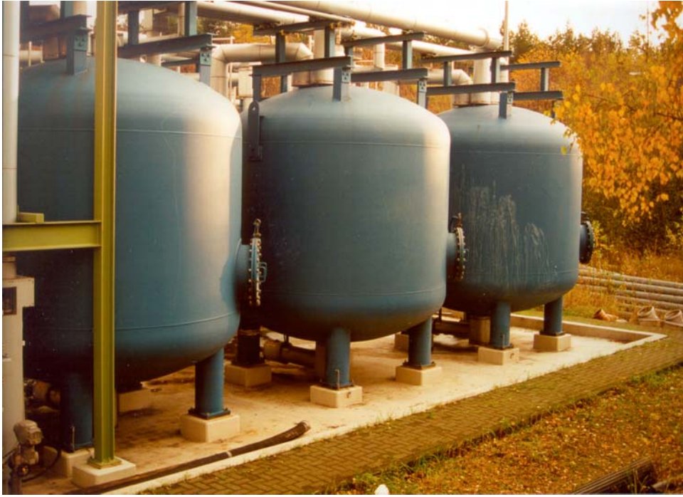
Plate 2.9: Typical external sequential GAC tank installation for polishing of biologically-pre-treated landfill leachate
