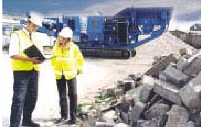
SEPA officers inspecting demolition waste at a construction site in Aberdeen
