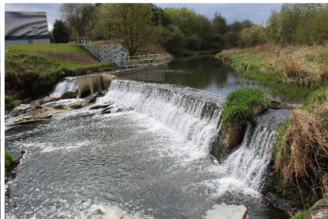
Kirkton Weir with fish pass installed
