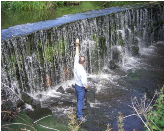
Sevenacres Weir before restoration
