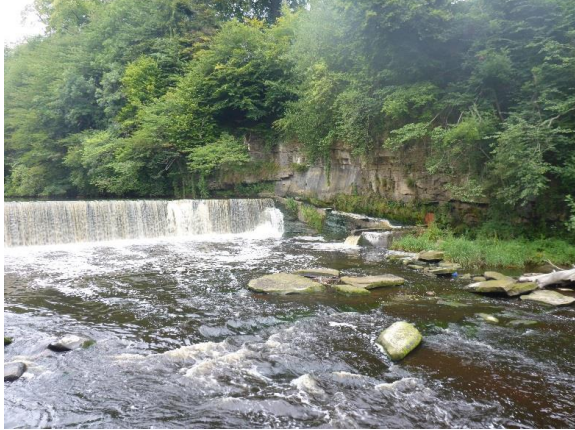
Fair A Fair Weir before works
