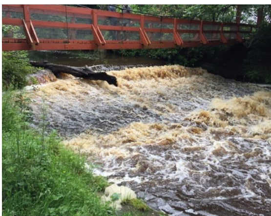
Garden Weir before restoration
