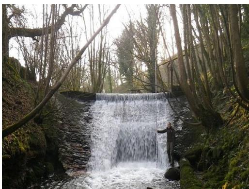
Tarff Creamery Weir before removal
