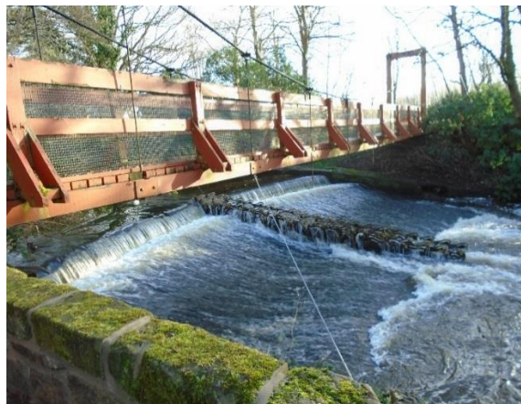
Garden Weir after fish pass installation (below bridge)
