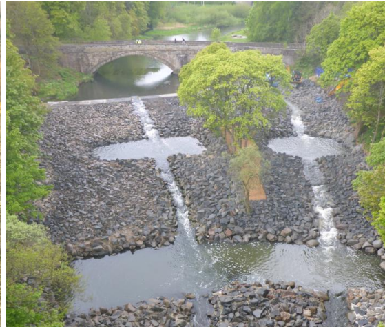
Howden Bridge Weir rock ramp installed
