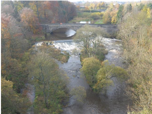
Howden Bridge Weir before works
