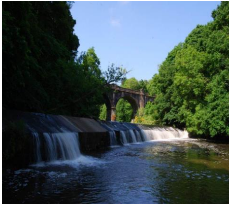
Ferniegair before fish pass installation
