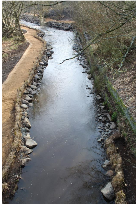
Rugby Club Wier bypass, after works
