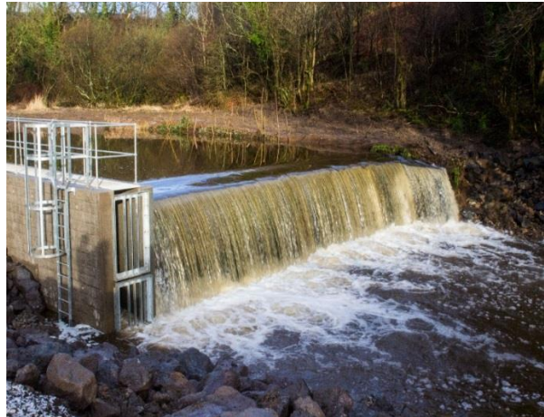
Sevenacres Weir after fish pass installation
