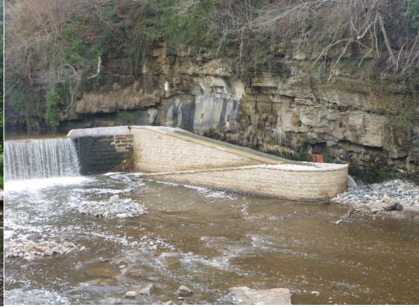
Fair A Fair with fish pass installed
