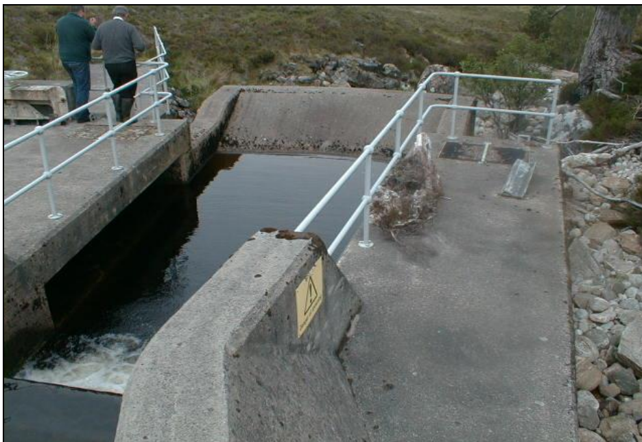
Picture 1: Scoop intake showing 'scoop' shaped central channel with side intakes. In high flow conditions the water continues over the crest of the intake and effectively scours the intake on every spill (photograph courtesy of Scottish & Southern Energy).
