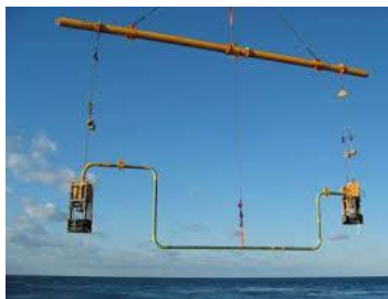
Jumper spool being deployed
