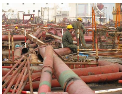
Topside metal being size reduced
