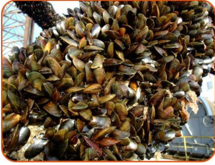
Marine growth on manifold protection support leg
