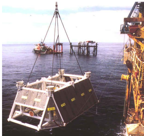
Subsea isolation valve being deployed
