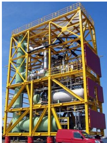
Modular operational produced/process water treatment system
