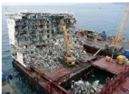
Topside metal module being decommissioned
